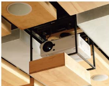
Around the horn: Behind the bar, Zachary shows David what's what on the all-powerful AMX touchpad (left). If you rent the place out for a corporate event, you can engage a Draper 119-inch retractable screen that drops down from the ceiling (top) and access an NEC DLP projector mounted in an Auton projector lift. Flanking the projector are two JBL in-ceiling speakers.
